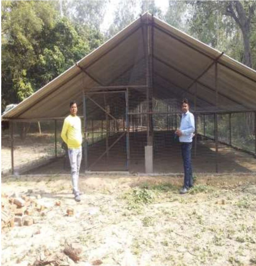
AT THE TIME OF WORK
